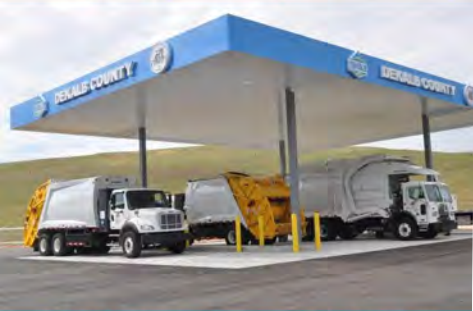
CNG Station – Seminole Road Landfill
