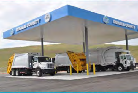
CNG Station – Seminole Road Landfill
