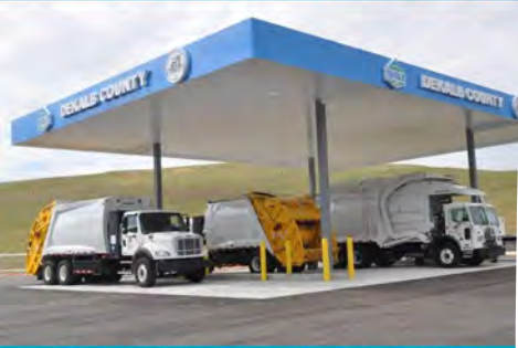
CNG Station – Seminole Road Landfill
