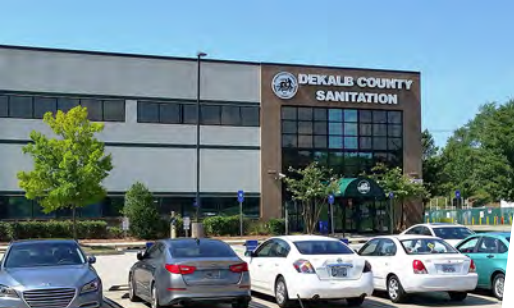
Sanitation Division Administrative Office
