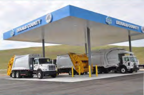
CNG Station – Seminole Road Landfill
