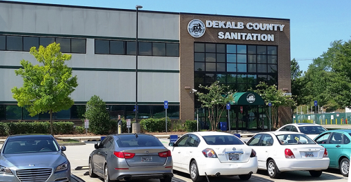
Sanitation Division Administrative Office
