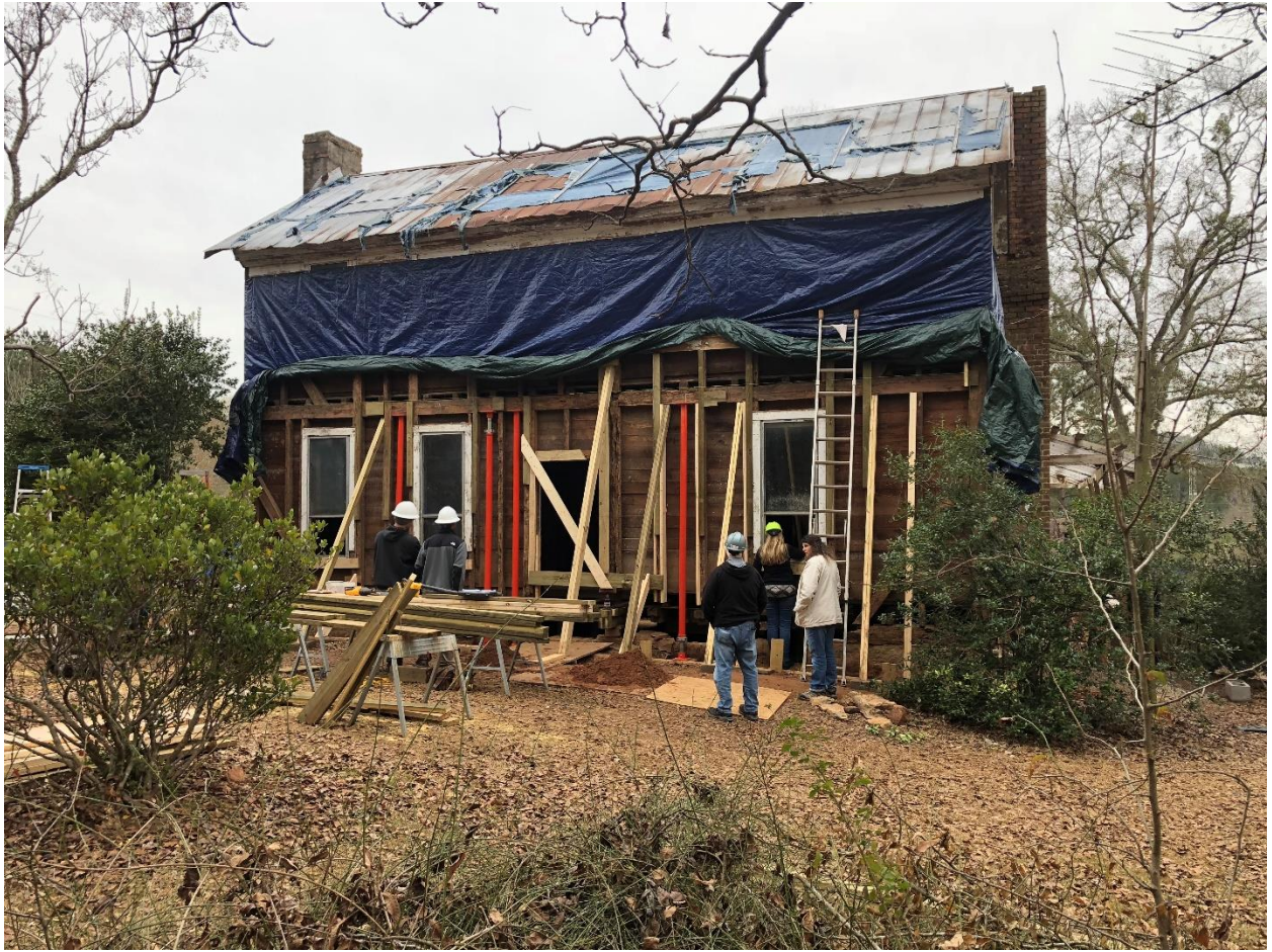
The Lyon Farmhouse, under construction in December 2018.
