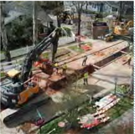
Upsize or replace 35 miles of small diameter sewer pipe
