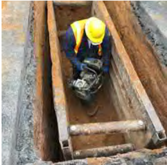
Perform 1,600 point repairs of localized pipe failures
