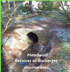
Storm Drain Receives excess water in rain events
