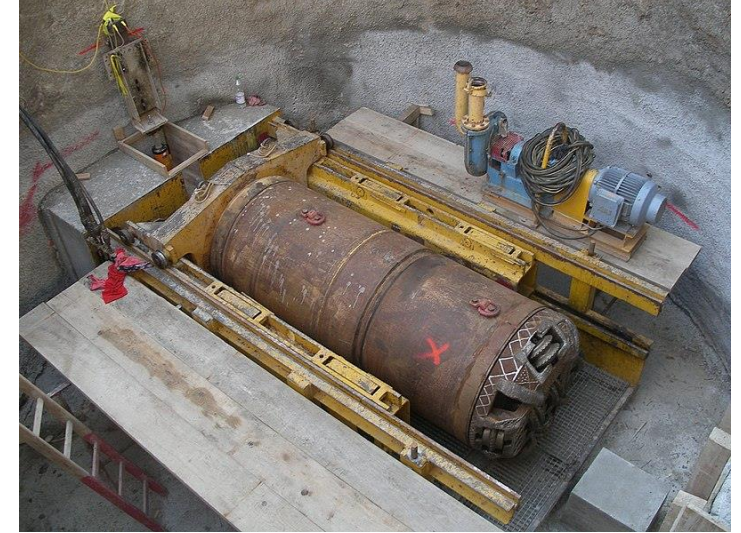
Jack and Bore and Micro Tunneling Under Major Highway/Interstate/GDOT Crossing
