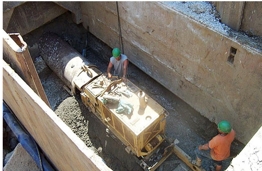
Jack and Bore and Micro Tunneling Under Major Highway/Interstate/GDOT Crossing
