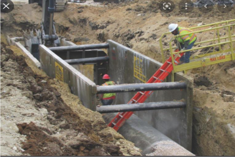
Open Trench Excavation – Majority of North Fork/ South Fork Peachtree Creek Trunk Sewer Upsize
