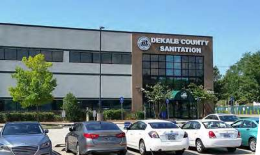
Sanitation Division Administrative Office
