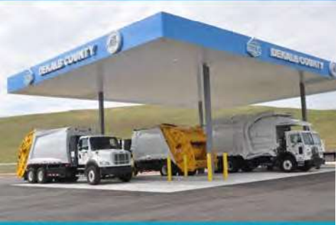
CNG Station – Seminole Road Landfill
