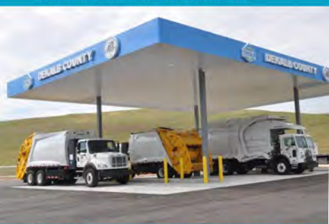
CNG Station – Seminole Road Landfill
