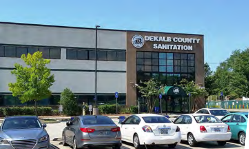
Sanitation Division Administrative Office
