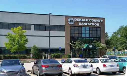
Sanitation Division Administrative Office
