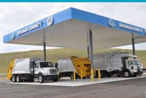
CNG Station - Seminole Road Landfill
