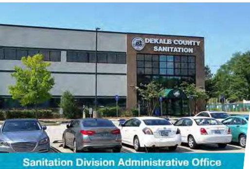
Sanitation Division Administrative Office
