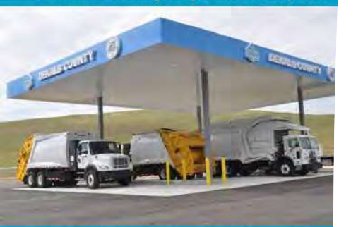
CNG Station - Seminole Road Landfill
