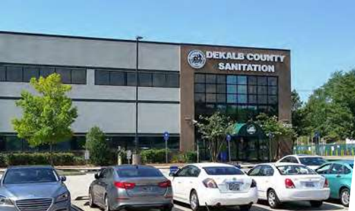
Sanitation Division Administrative Office
