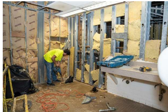
Flat Shoals Library Renovation underway
