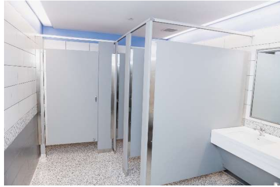
Completed renovation at Decatur Library
