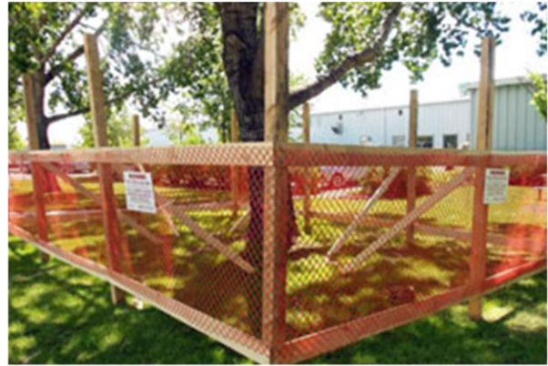
Compliant Tree Save Fencing Can be any sturdy material, t-posts, wood etc.
