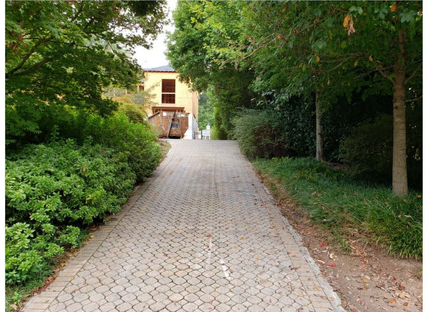
View of Out-Building From the Sidewalk
