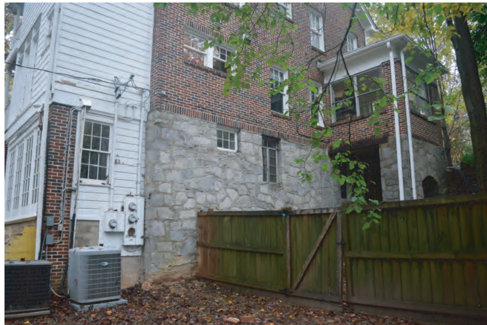
View of rear corner of house from northeast. Shows non-historic addition from period when home was being used as a multi-family residential triplex.
