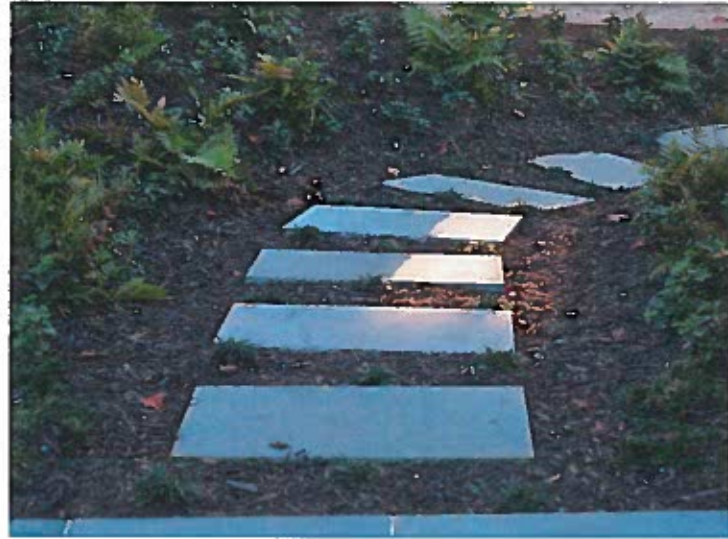
Bluestone steppers with planted joints
