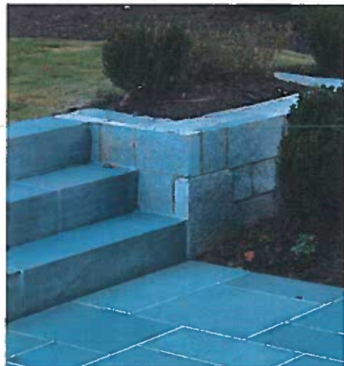
Granite ashlar retaining wall
