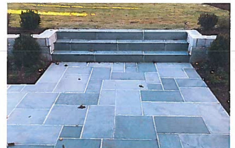
Solid slab bluestone stairs with granite retaining wall
