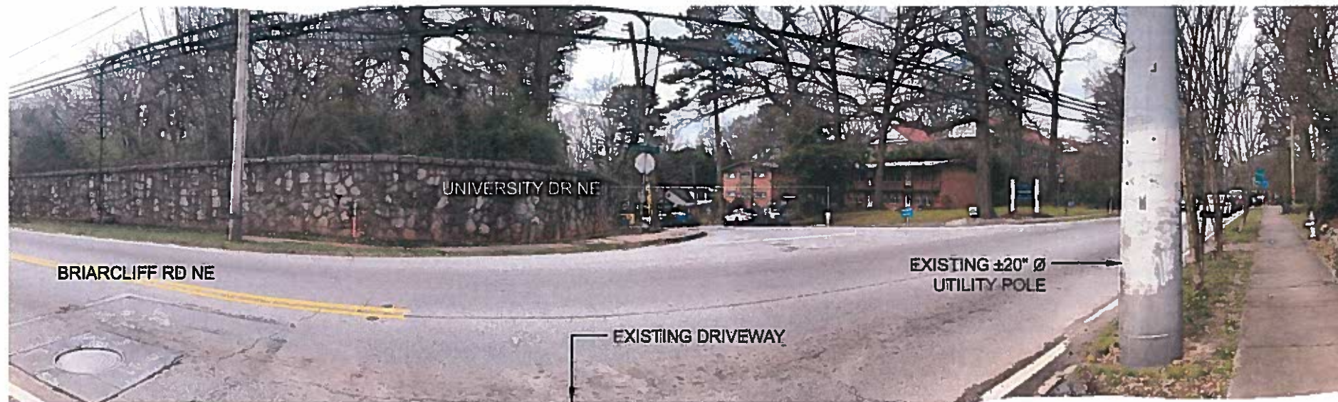
EXISTING DRIVEWAY EXIT TO BRIARCLIFF ROAD PHOTO TAKEN 5 FT FROM EDGE OF ROADWAY
