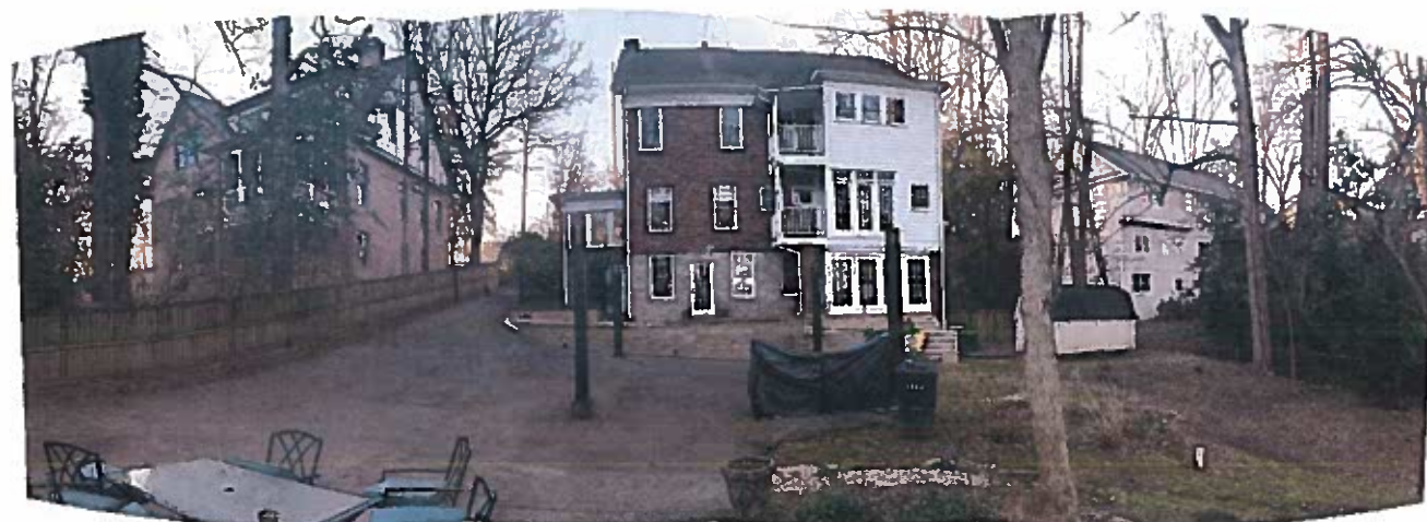
NORTHWEST VIEW, BACK OF RESIDENCE
