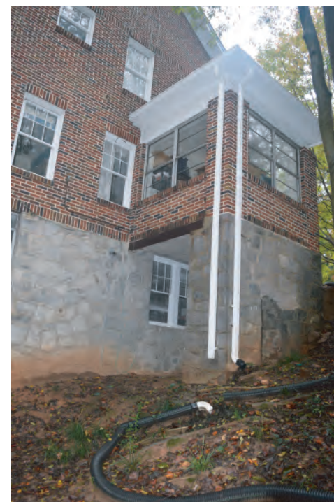
View of northeast elevation. Porch was closed in at some point with metal jalousie windows.
