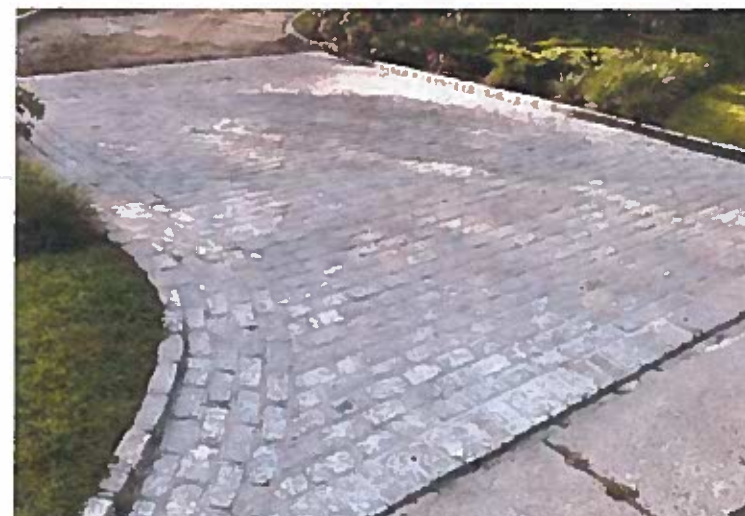
Cobblestone paving - running bond
