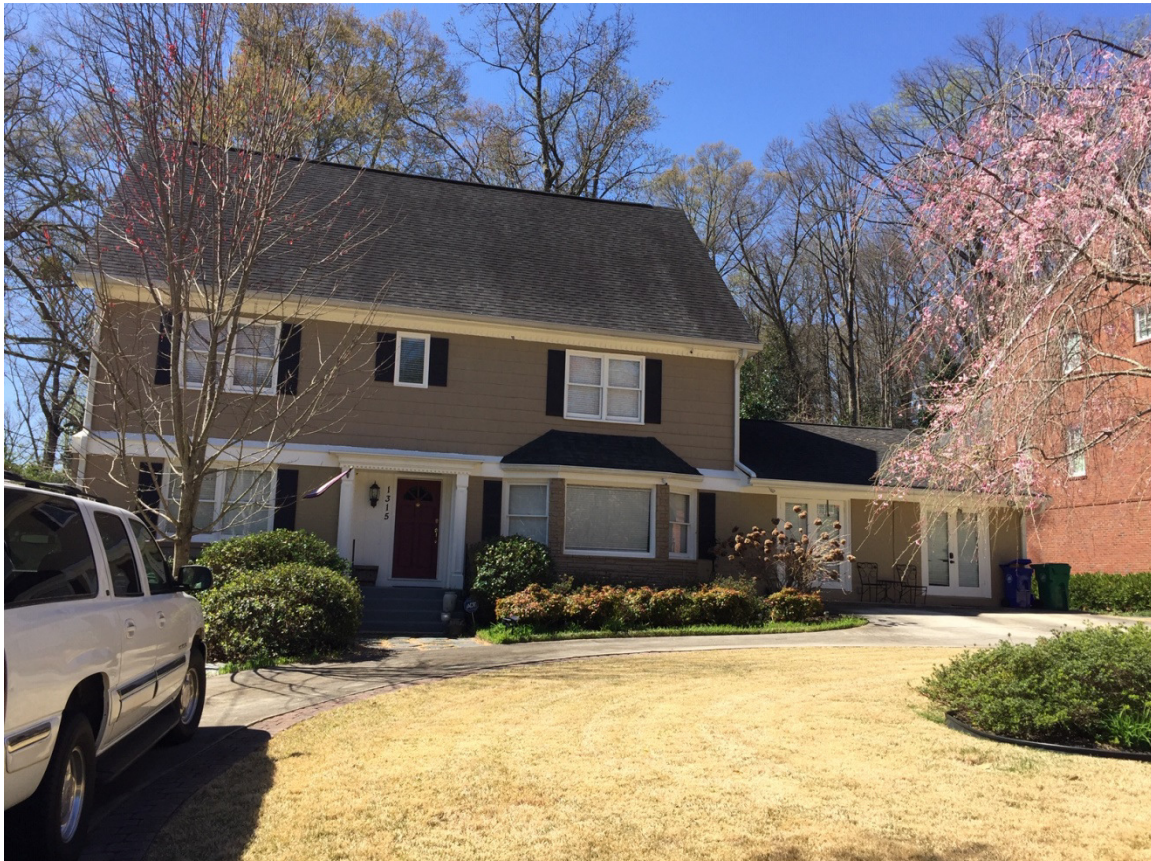
View of Front Elevation (small window to receive frosted sashes)
