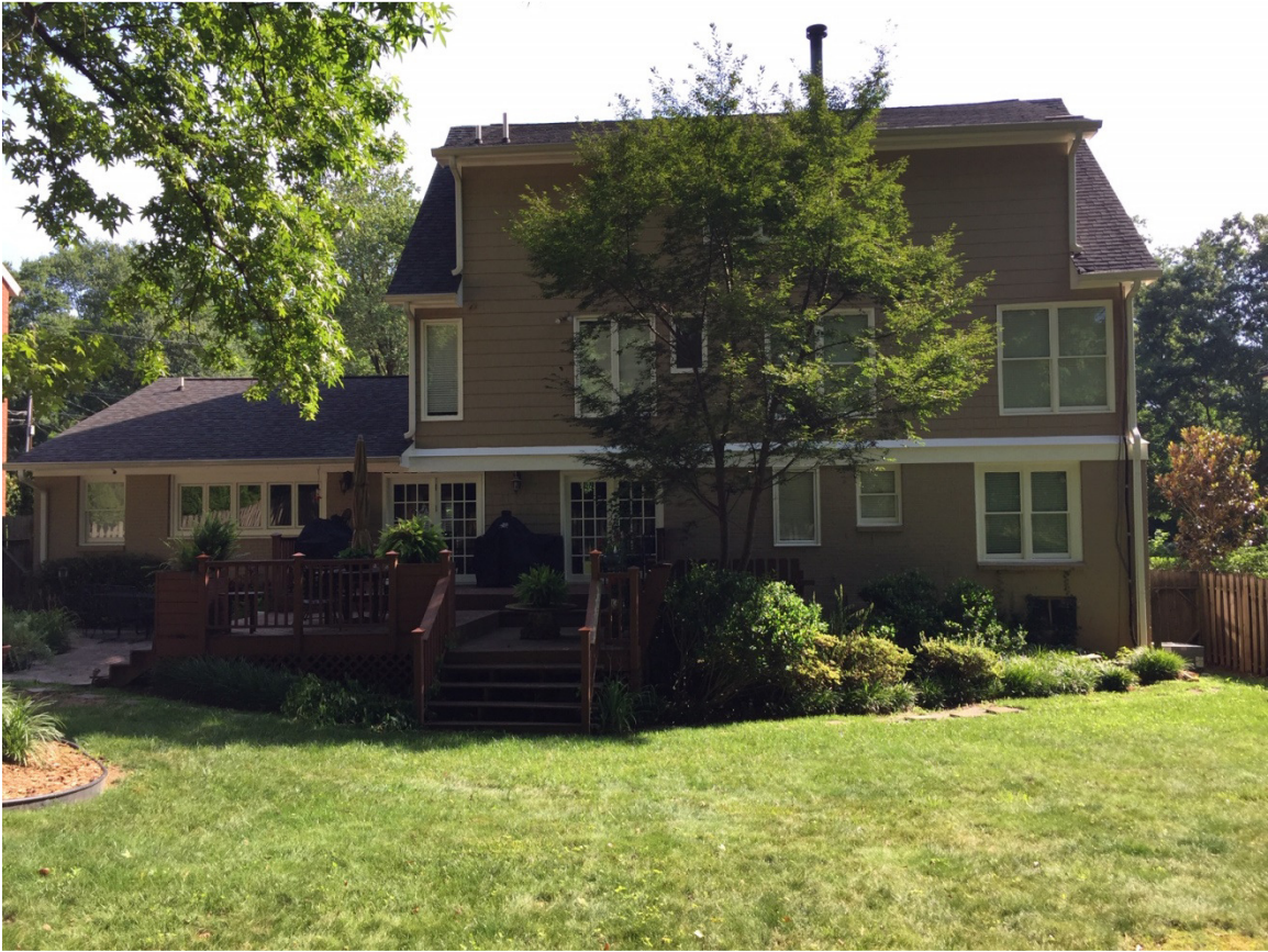
Rear View - Demo middle pair of wood windows and shift ex. small window over (infill with cedar shakes to match ex)
