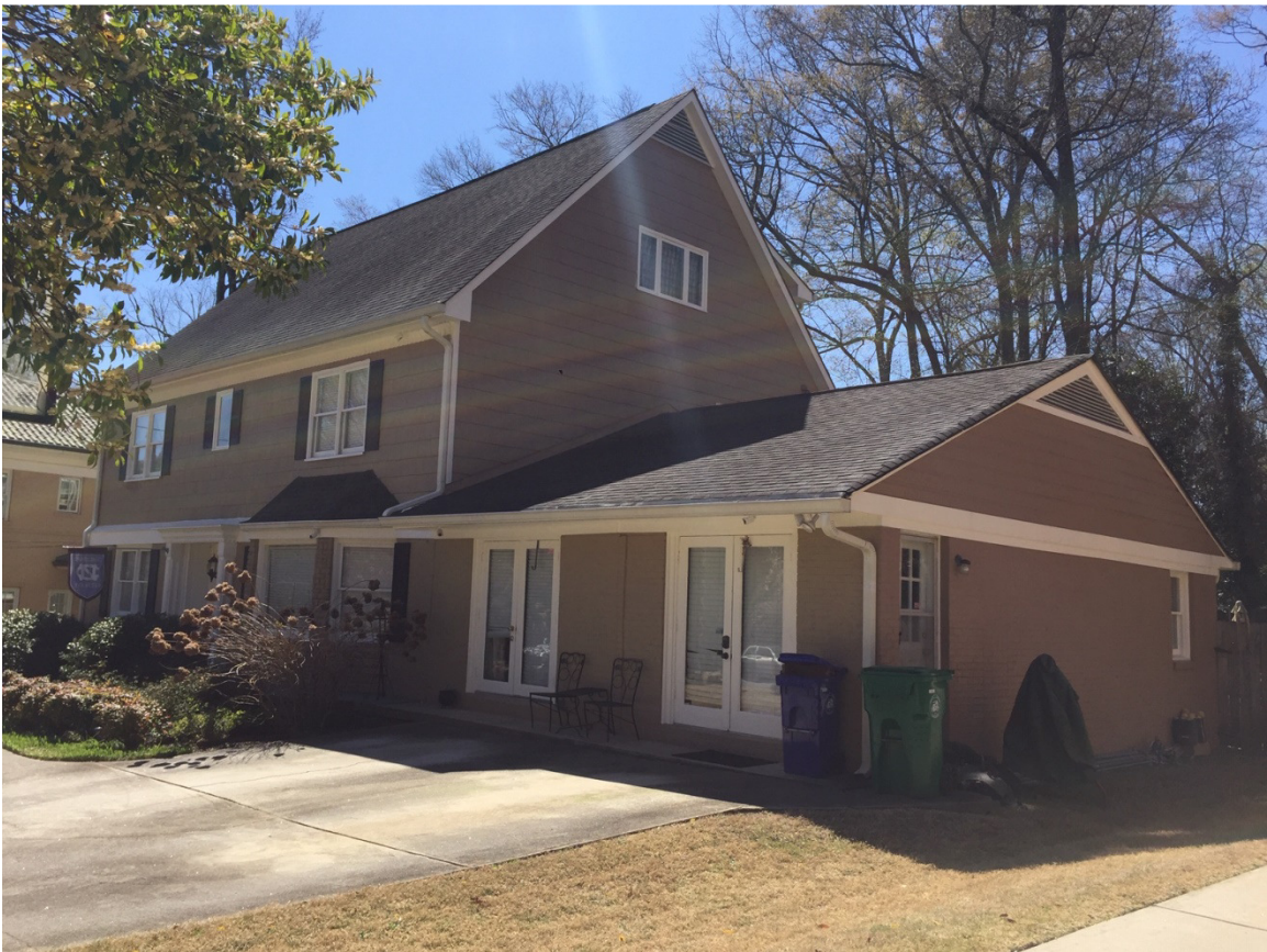
View from Right-of-Way from Right Side of Street (NW) – Door on Side of Garage to be changed to a window with brick infill below
