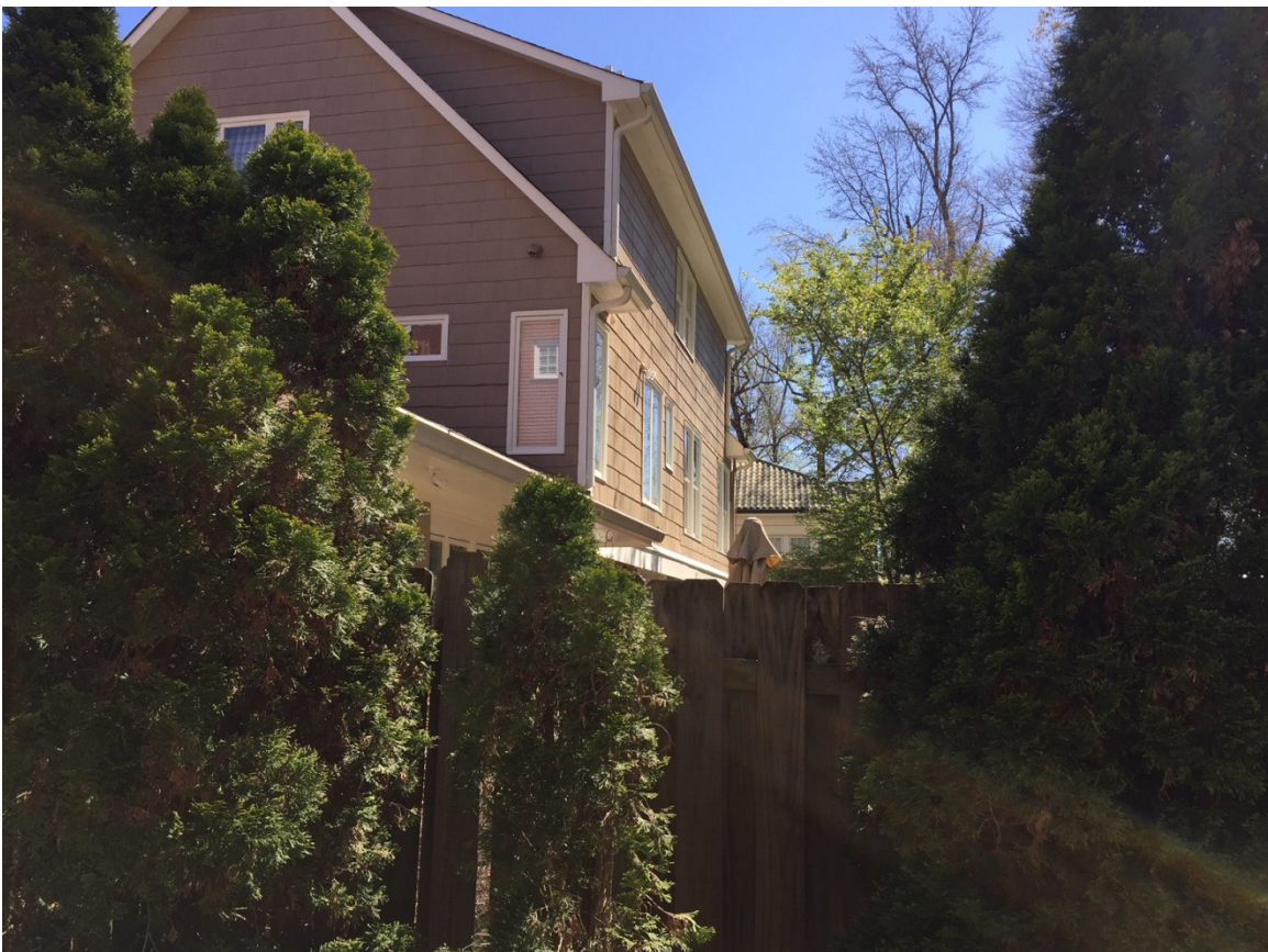
View of SW rear corner (corner windows to be removed with cedar shake infill)
