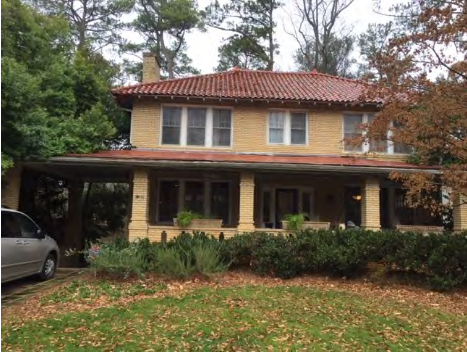
1388 Cornell Rd. Roof and gutter to be replaced is over porch and porte cochere.
