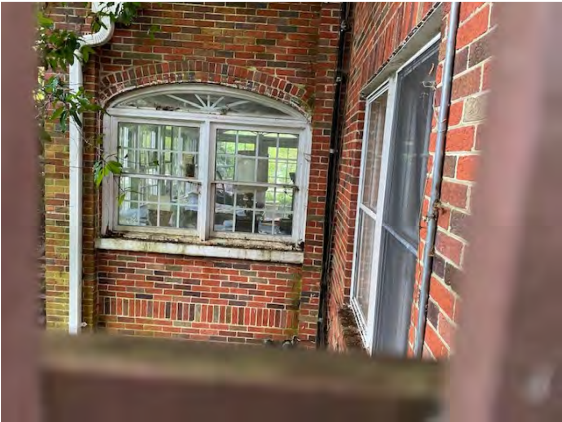
Sample of rotten sill to be replaced
