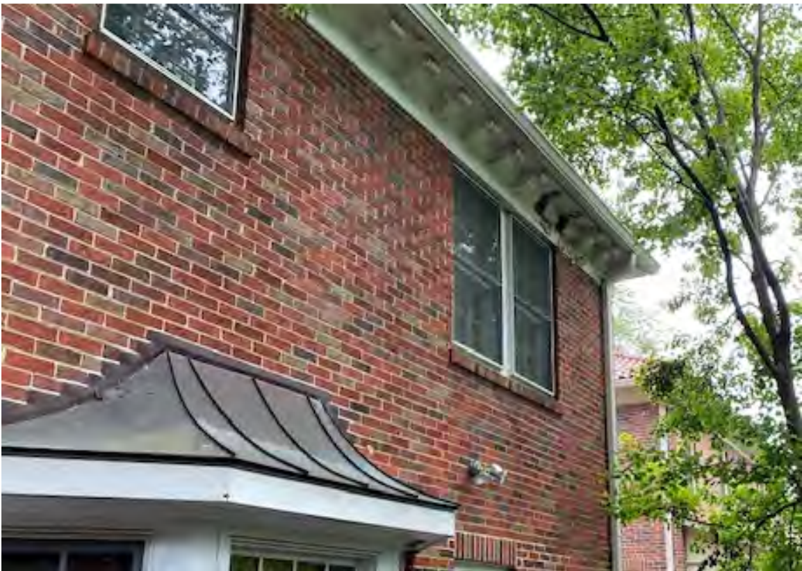
Existing soffit & corbels in need of restoration
