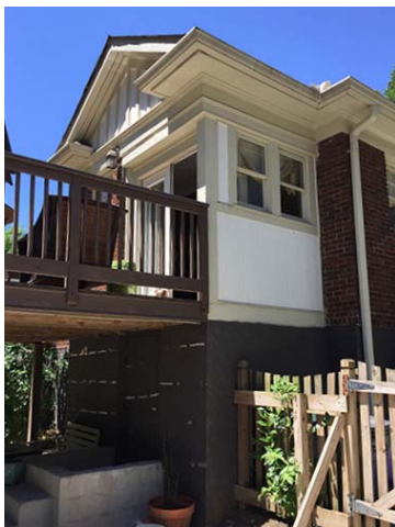
Existing side elevation showing rear addition
