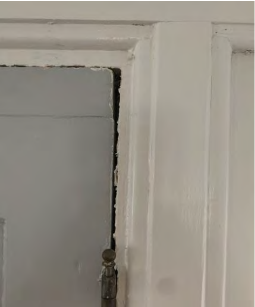
Poor Alignment, Layers Upon Layers of Old Paint
