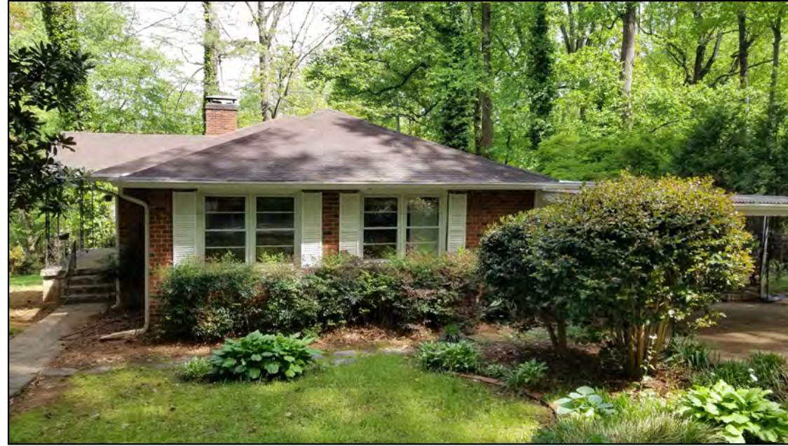
right side of existing home
