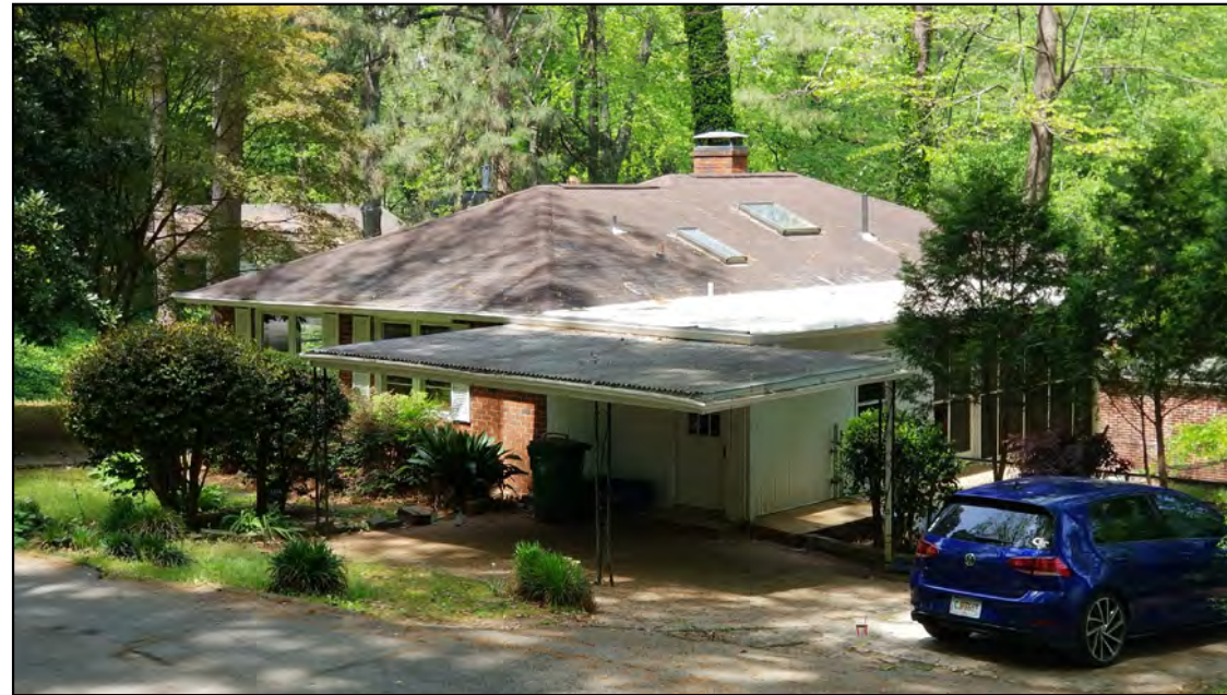
existing car-port and non-conforming addition which are to be removed
