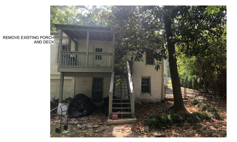
REPLACE EXISTING DOUBLE HUNG WINDOWS WITH ALUMINAM CLAD DOUBLE HUNG WOOD WINDOWS WITH 6 OVER 6 SIMULATED INSTALL NEW DOUBLE CASEMENT DIVIDED LITE PATTERN ALUMINUM CLAD WOOD WINDOW
