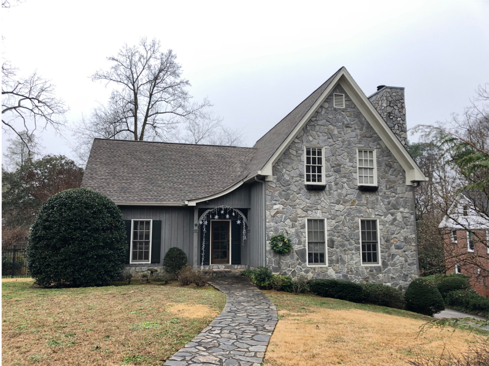
South Elevation - Front of house from Ponce De Leon Manor
