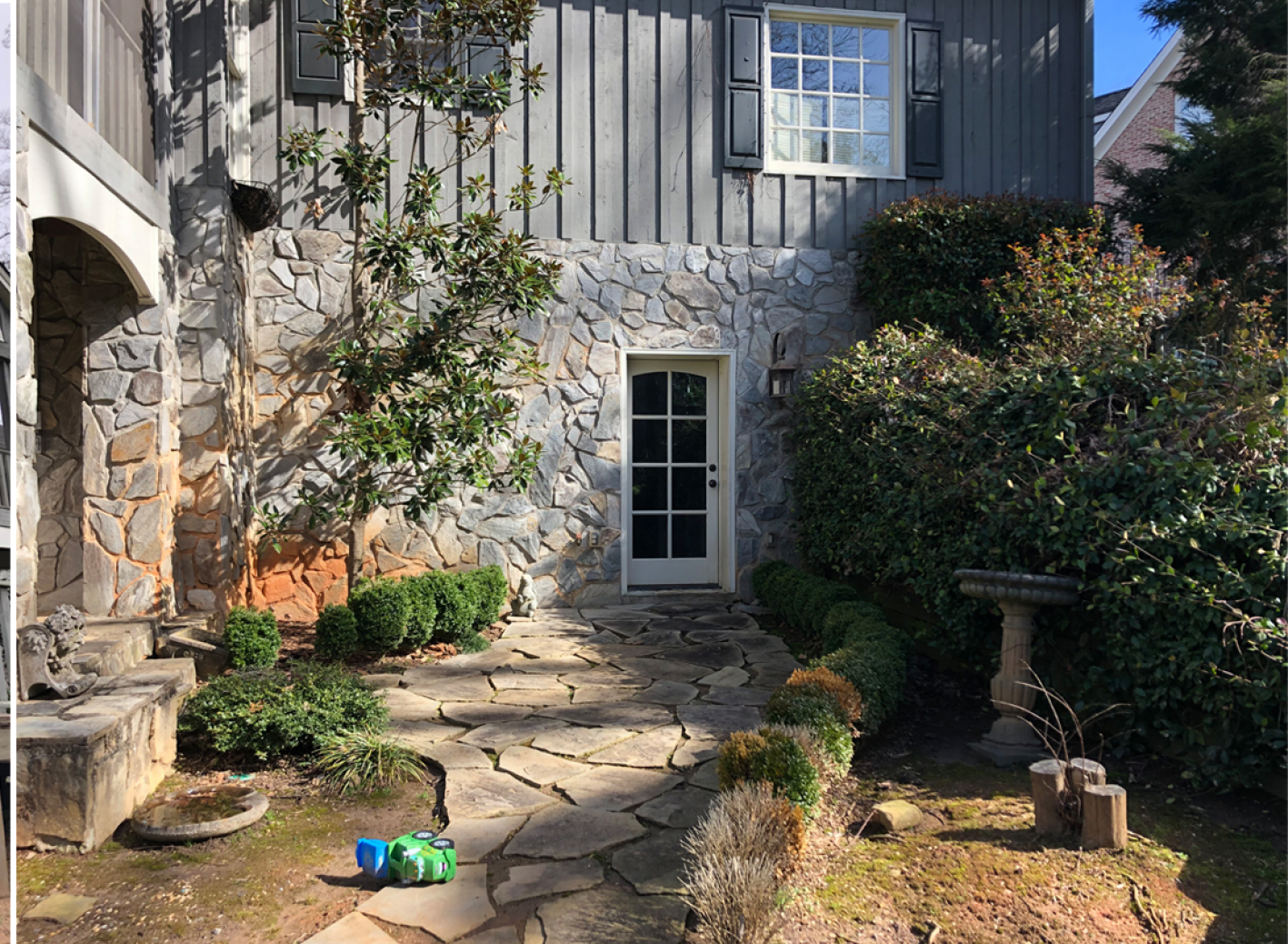
North Elevation - View of paved path to the basement
