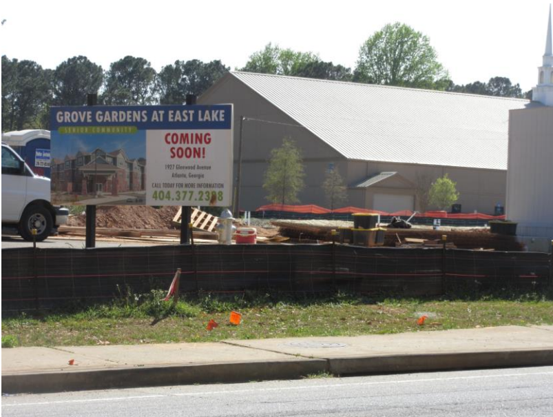
Senior Living Facility Under Construction Across the street
