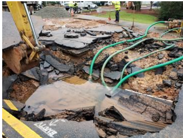
DeKalb Watershed crews repair a damaged 20-inch water main.
