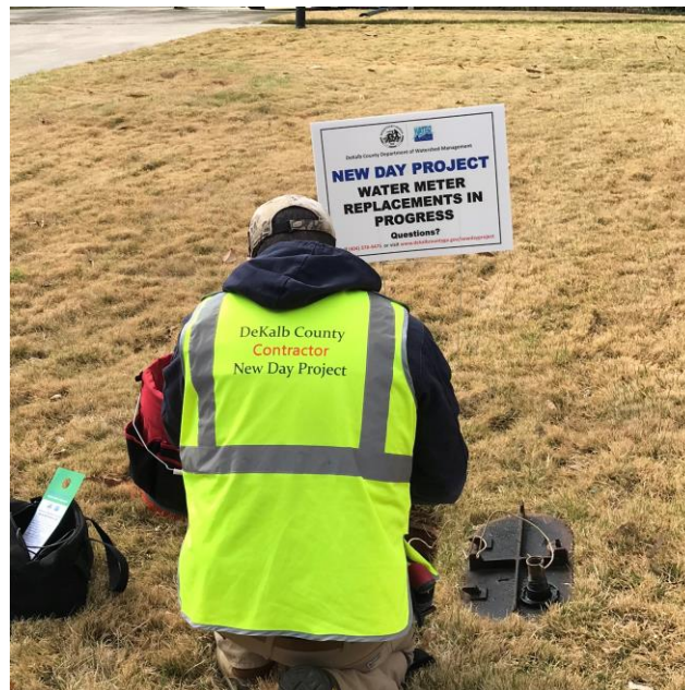
Contractor installs new water meter.
