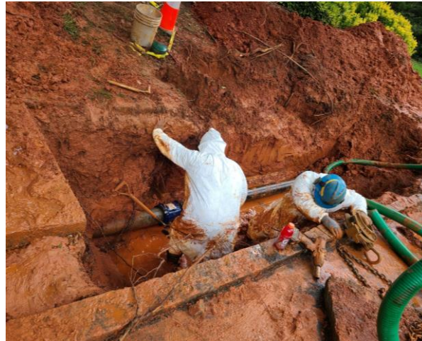
DeKalb County watershed crew completes repair.
