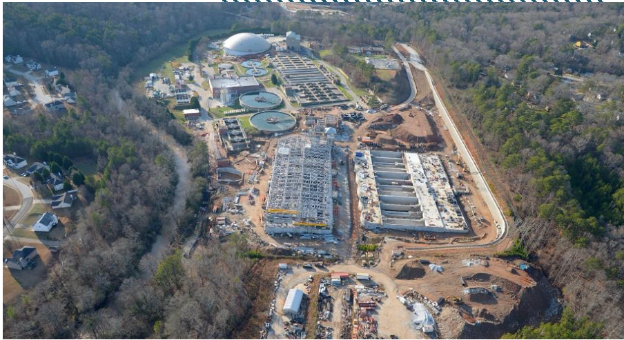
^ Snapfinger Wastewater Treatment Plant
