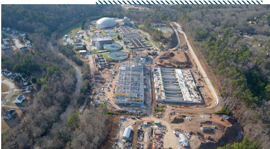
^ Snapfinger Wastewater Treatment Plant
