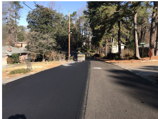
Crews have paved more than 180 roads in DeKalb through the SPLOST program.
